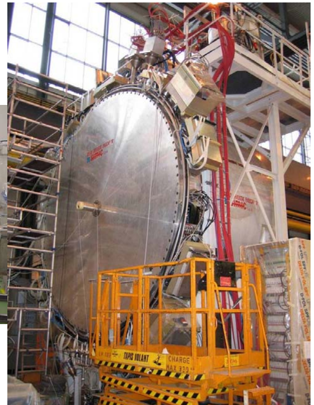
End-Cap A during the surface cold tests
